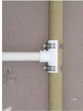
The polarity of the dipoles must be consistent, so make the connection to the top element of each dipole with the coax center conductor and the coax shield to the bottom element.
