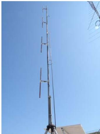
For omni directional coverage arrange the dipoles around the mast so they each cover a compass heading 90 degrees apart from each other. For example, if the top element faces north, the next one down will face east, next below that will face south and the bottom dipole will face west. You can aim the top dipole in the direction of your weakest signals.
